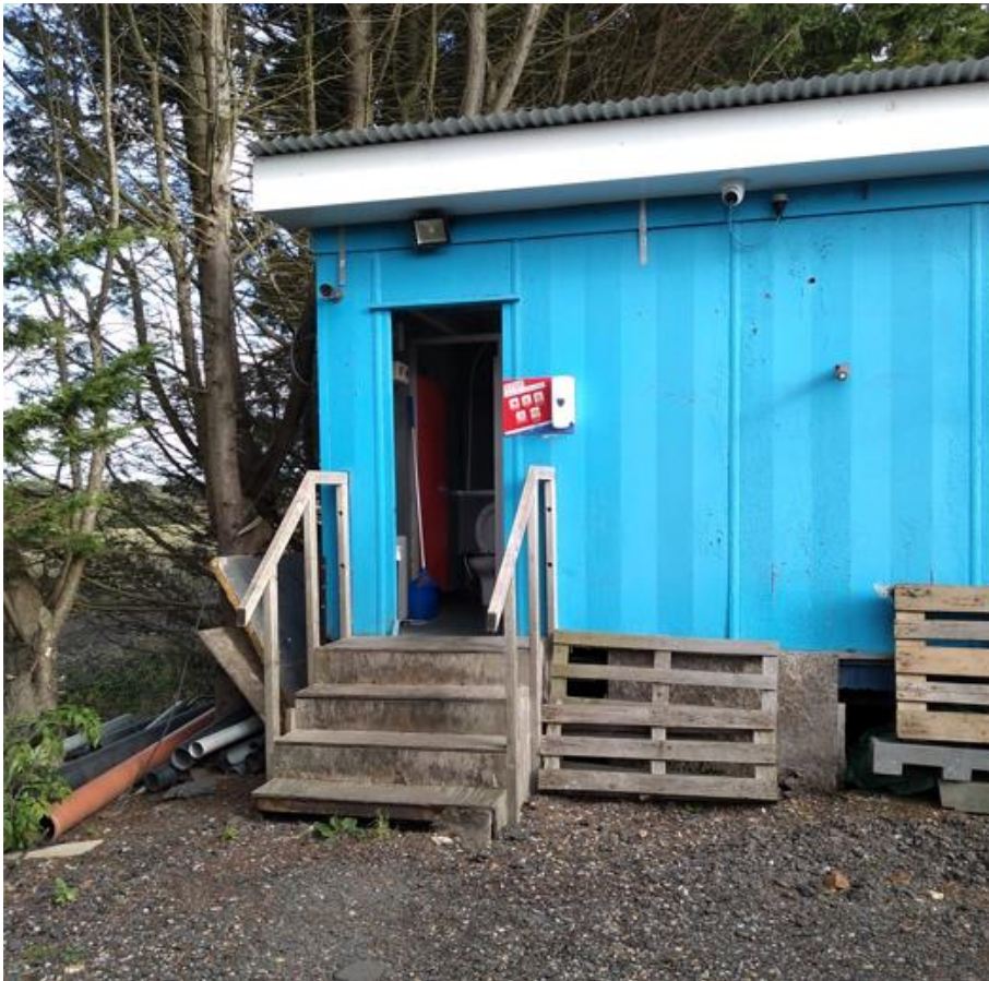
Figure 3 – toilet and shower units
